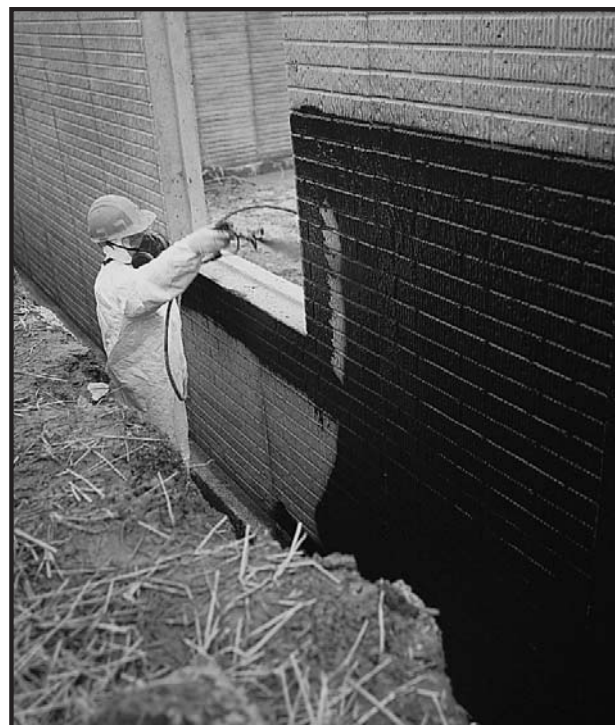
MULSEAL dampproofing is spray-applied for seamless coverage of foundation walls.
